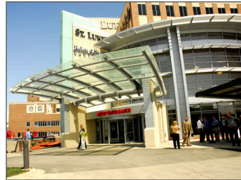
St. Luke's Hospital
