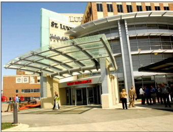
St. Luke's Hospital
